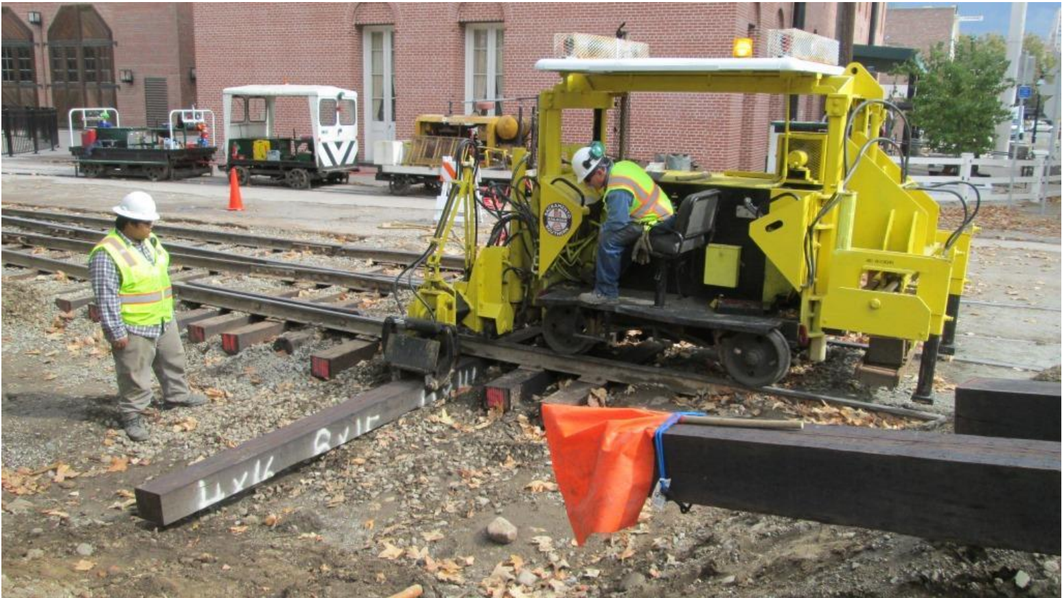
Then get it inserted under the rails
