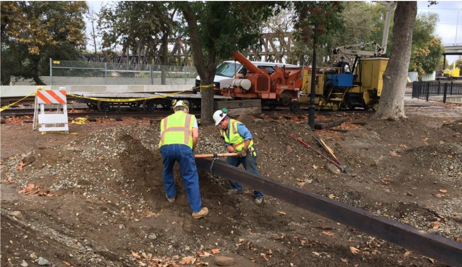
Clem and Joe manhandle a new tie into position...
