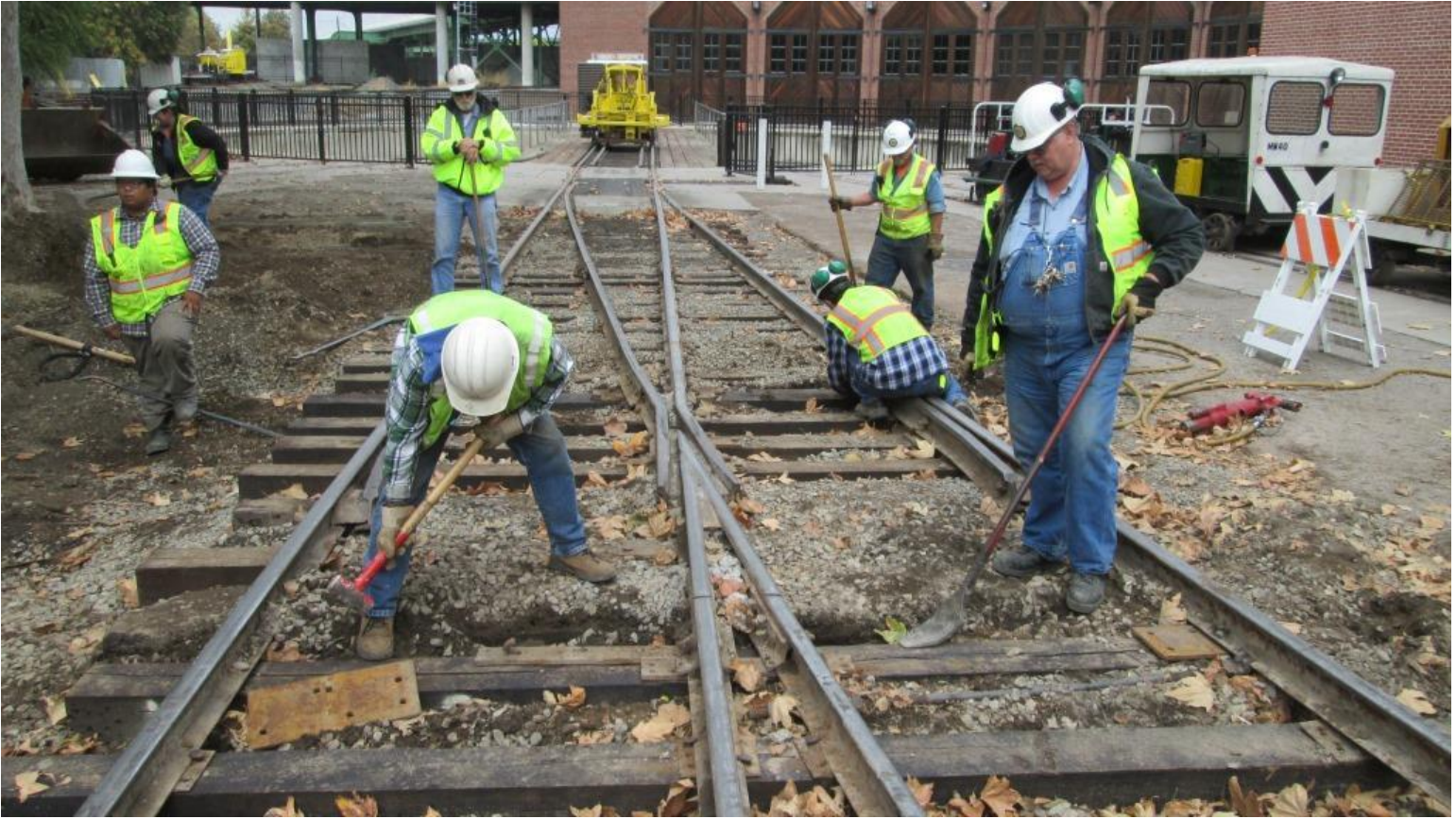
Mike M. uses a little gentle persuasion to get the frog-plate under the rails
