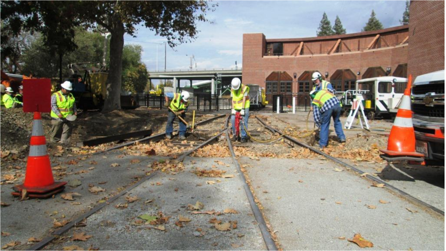
Under the protection of a "red-flag", the Team continues nipping and spiking
