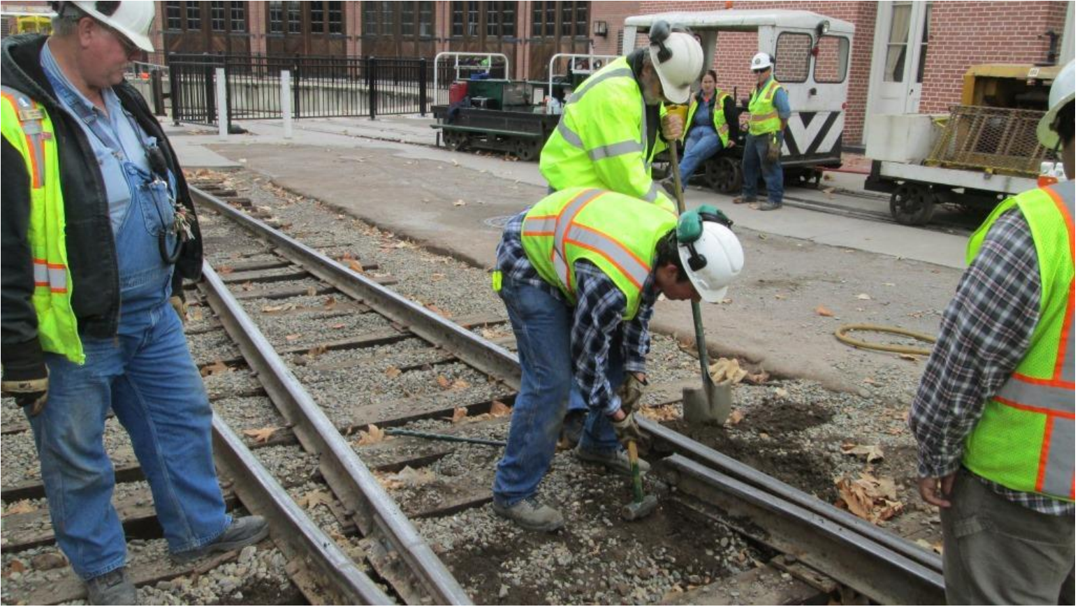
Weston works to pry an old plate loose
