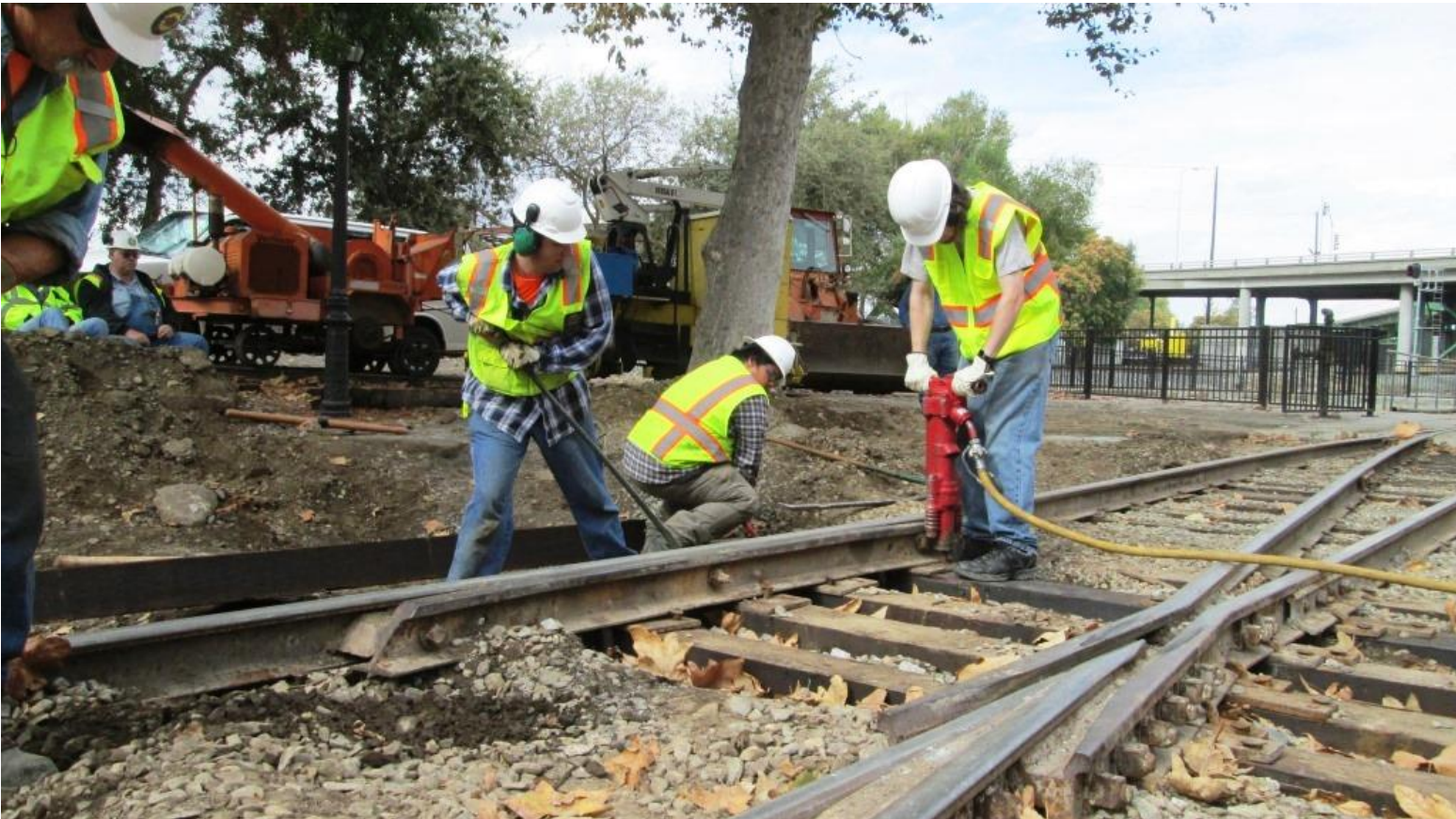
Weston and Anthony nip-up the switch-tie as Matt drive spikes with the pneumatic spike-driver
