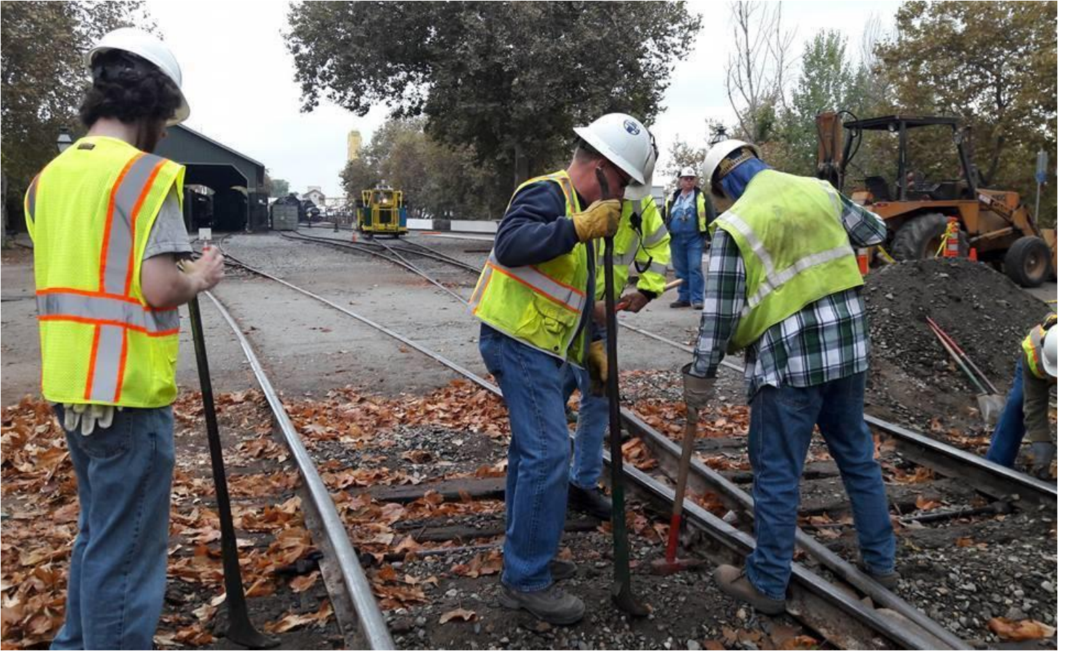
Ed and Mike M. work-loose rust-welded spikes with the spike-lifter
