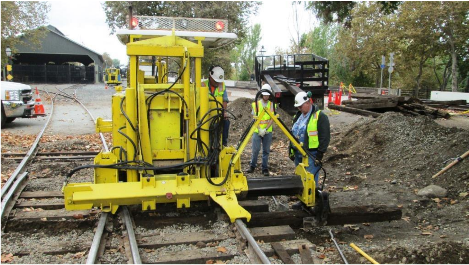
Joe pulls out a bad tie with the Jackson 125 tie-exchanger
