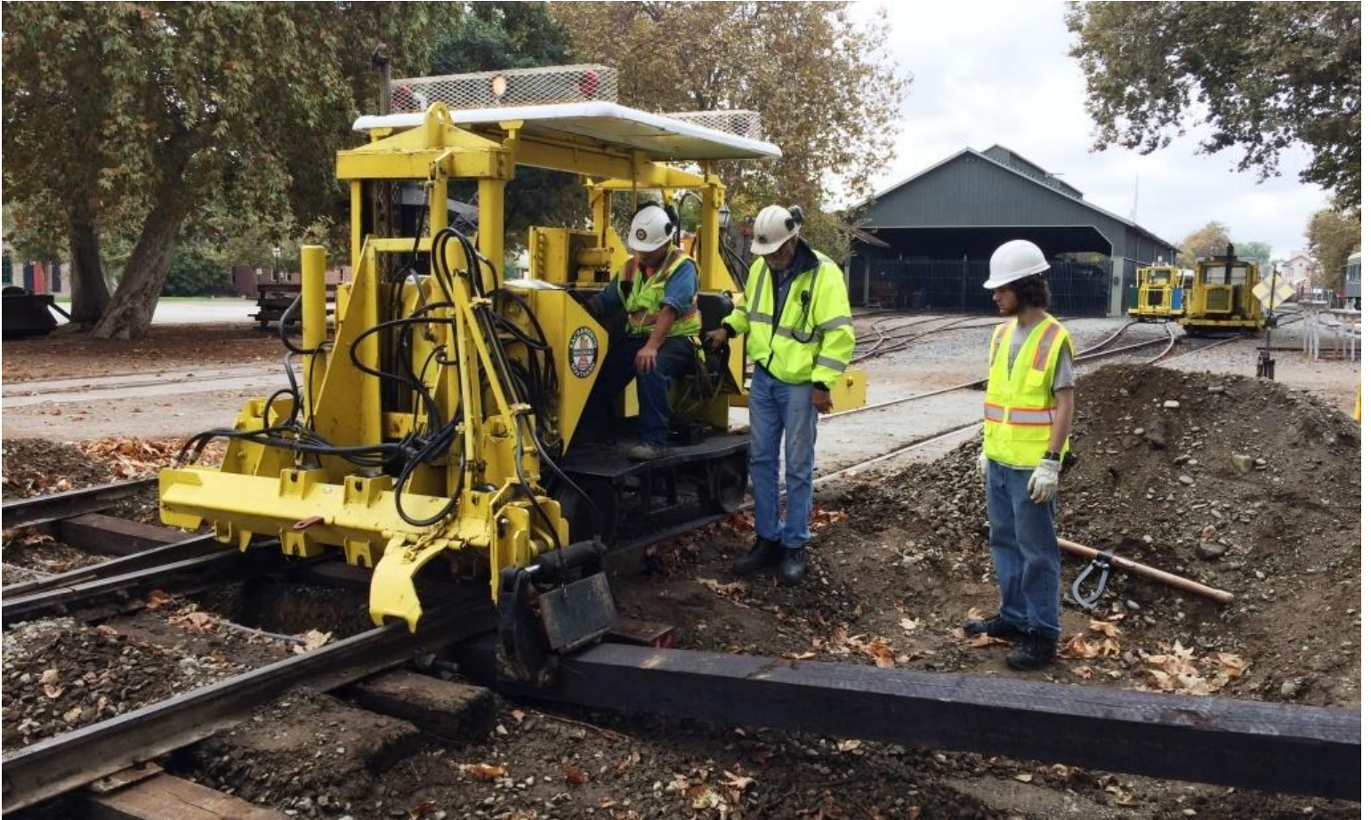
...The 15-foot long tie is then inserted under the rails
