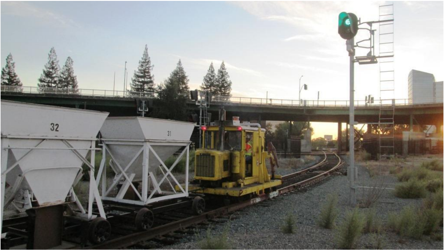
With signal indication showing green, Mike and Matt in the Kalamazoo pull the hopper-cars over the UP Main
