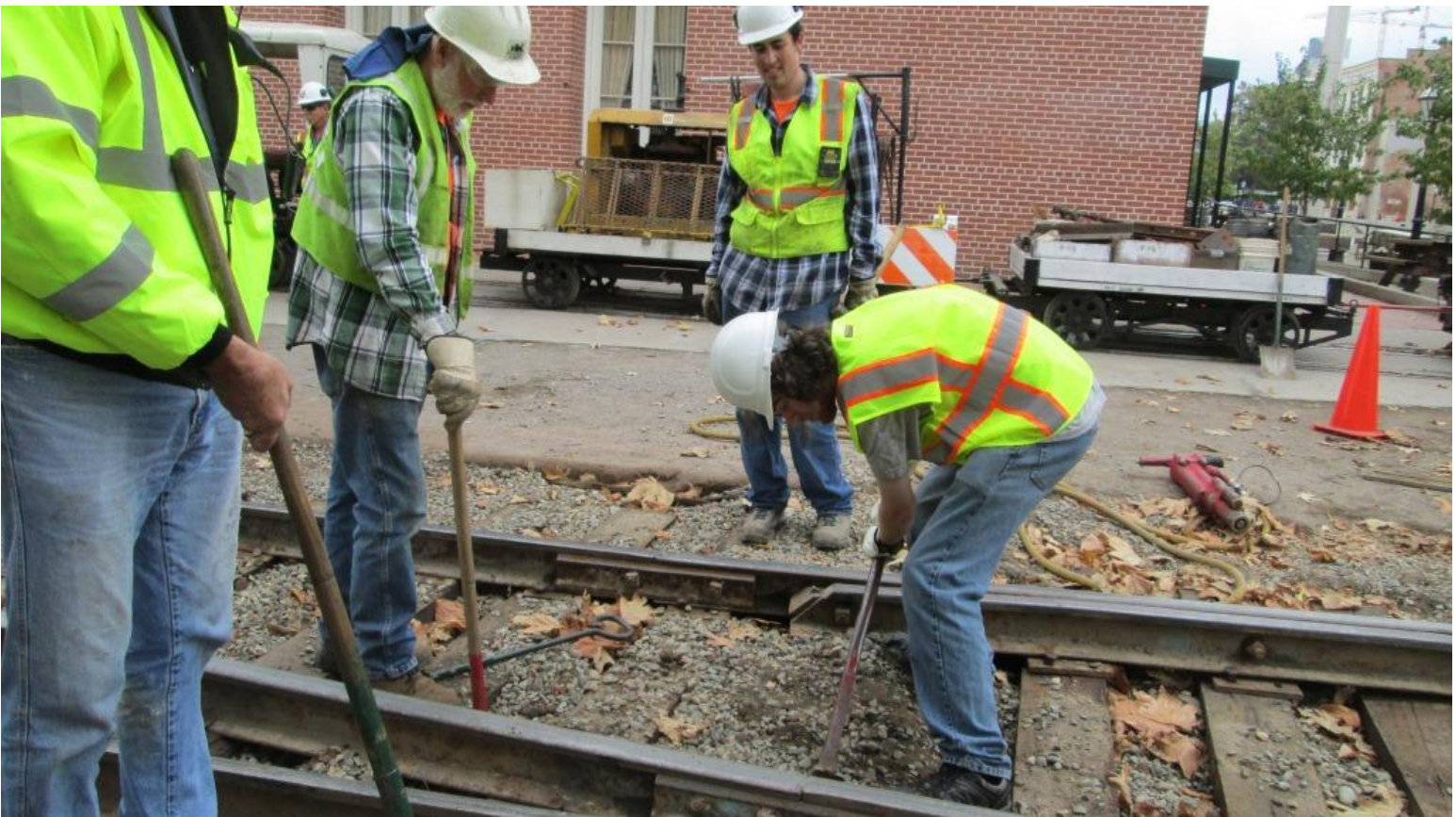
Matt uses a claw-bar to pull-out a rust-welded spike
