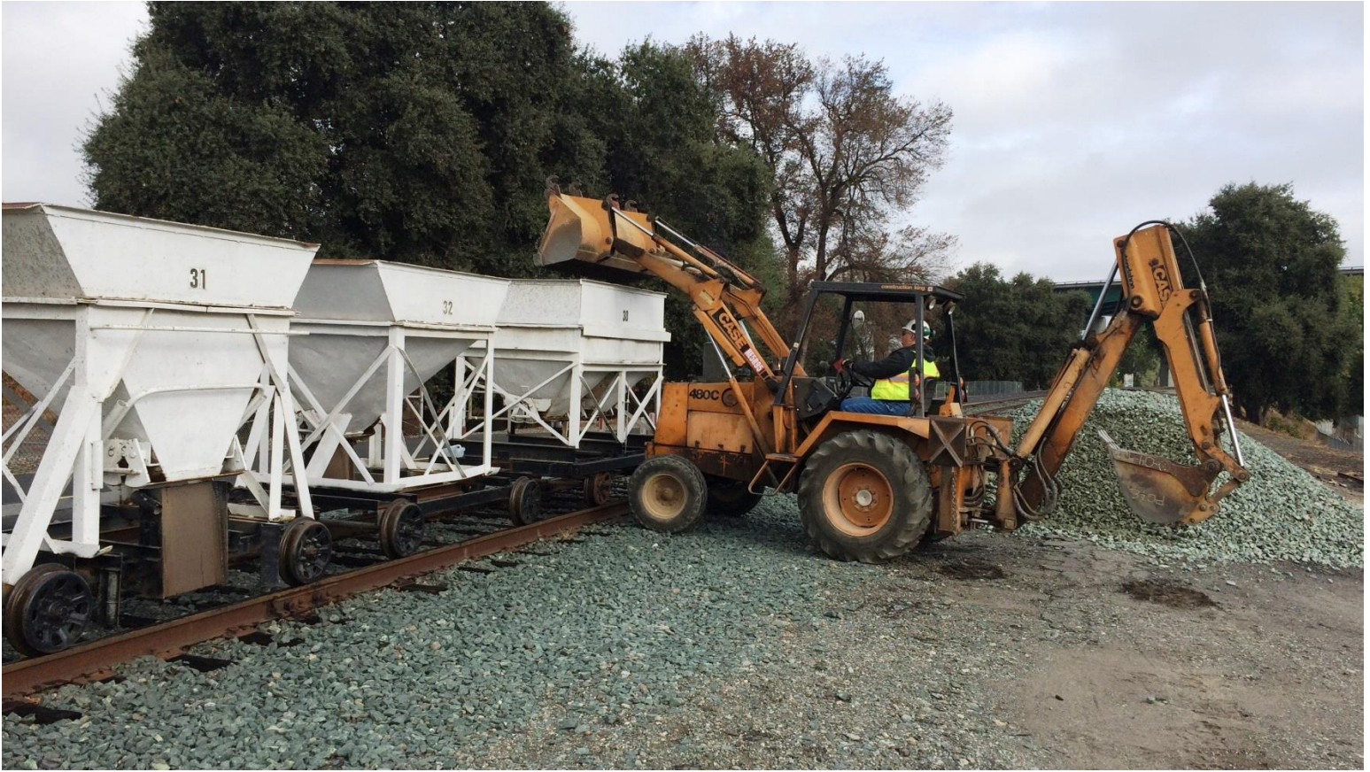
Chris loads ballast-rock into the hopper-cars
